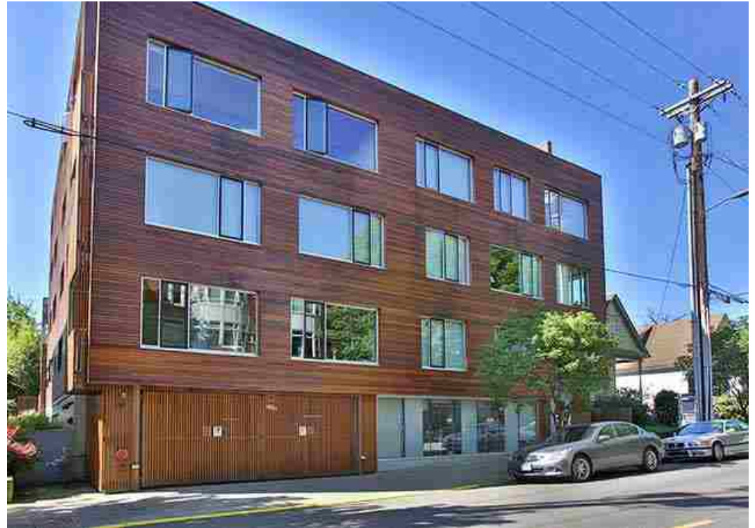
Fig. 3.19 Photograph of Thurman Street Lofts
