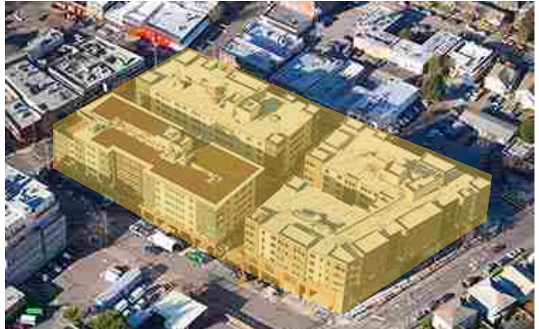
Fig. 2.25 Greenlake Village, aerial photo
