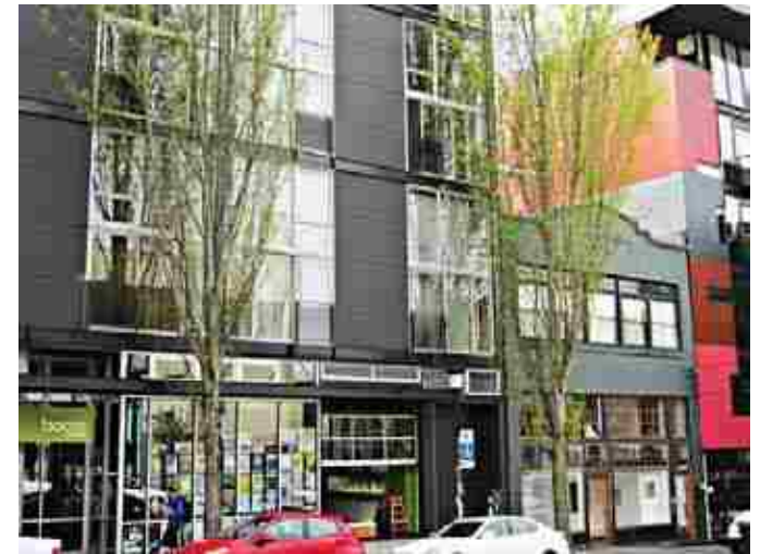
Fig. 2.18-19 New and old structures coexist on Capitol Hill, Seattle.
