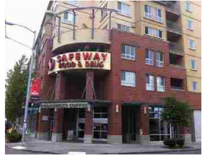
Fig. 2.43 Photograph of Summit at Madison Park, facing southeast
