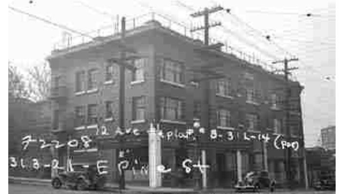
Fig. 2.33 Timkin Roller Bearing Building, ca. 1937
