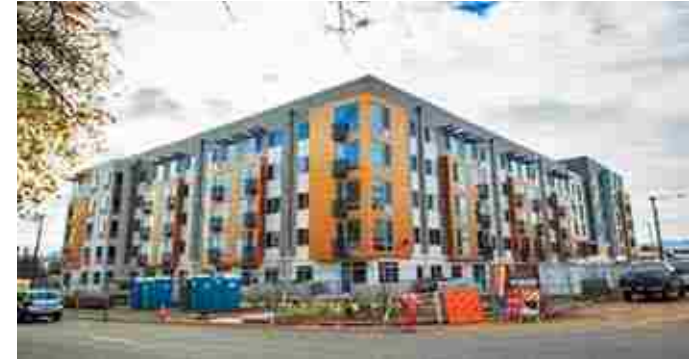
Fig. 2.48 Photograph of the Prescott, facing southwest
