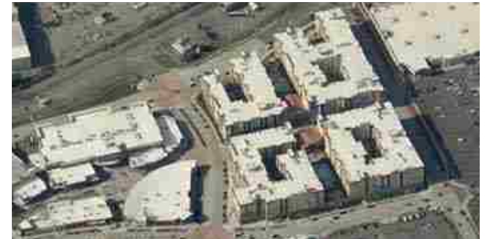
Fig. 3.2-3 The Landing, Renton Washington. This type of development has provoked criticism as ‘instant urbanism’ and lead to calls for parcelization to create more diversity and prevent simultaneous obsolescence.
